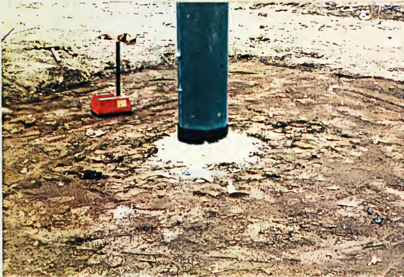
A22: CPN DENSITY PROBE USED TO CHECK DENSITY OF EACH LIFT
